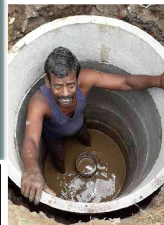
Varsha Rakshita: Rainwater Harvesting well, work in progress
